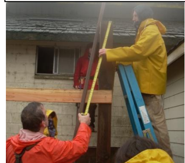
The YouthBuild crew on the job.
